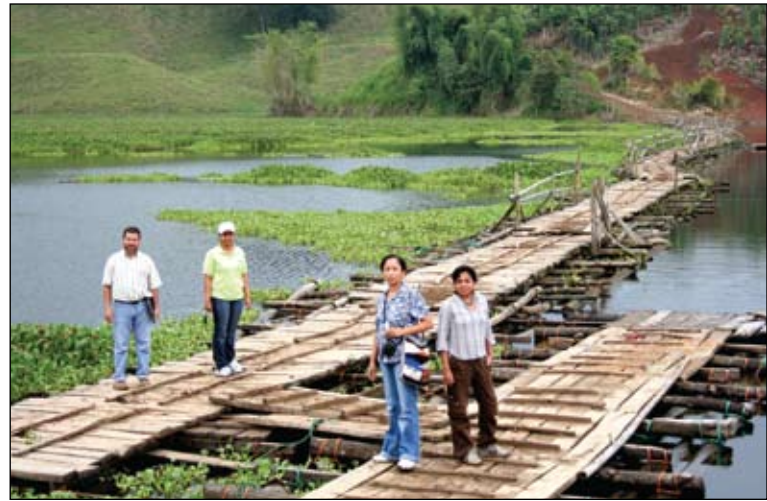
Picture: artisanal crossing bridge built by private individuals in the Manga del Cura territory
